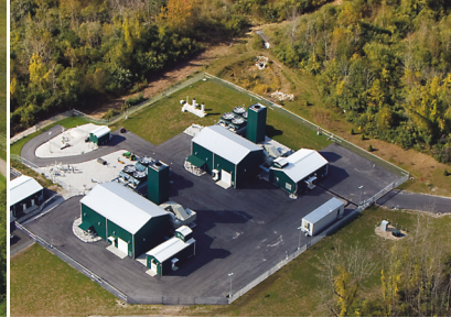
Brookfield, CT Compressor Station
