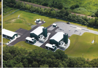
Milford, CT Compressor Station
