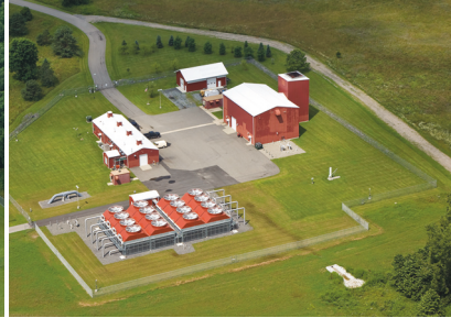
Dover, NY Compressor Station
