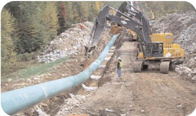
Newtown, CT: A section of the pipeline loop is placed in ditch.
