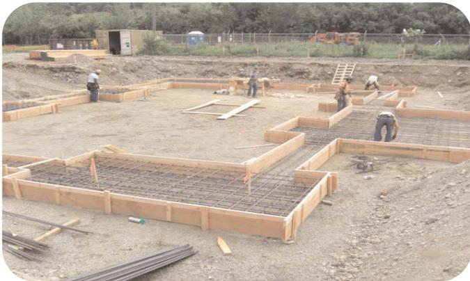
Milford, CT: Laying out the foundation forms for the new compressor station.
