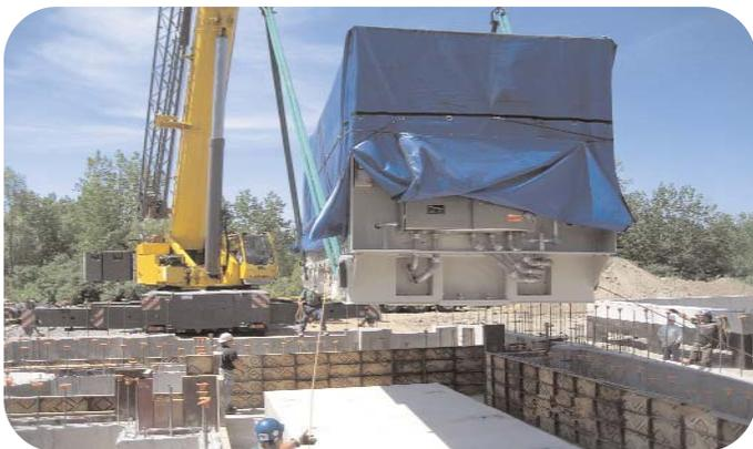
Brookfield, CT: Positioning the compressor unit onto its foundation within the station building.
