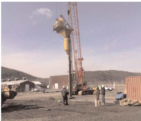
Construction activities in Dover, NY - ground reinforcement & soil stabilization
