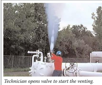
*Technician opens valve to start the venting.*
