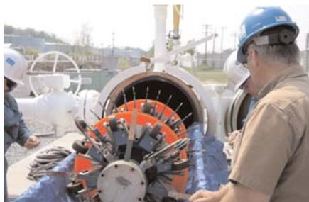
Insertion of pig into launcher
